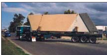
Panels in storage at precaster's yard awaiting delivery (above) and a 12.6 m x 3 m precast panel being transported from factory (left)
