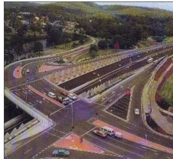
Elevation of multi-hued panels after erection (above) and an aerial view of Nerang-Broadbeach Road featuring some 362 precast noise barrier panels (right)
