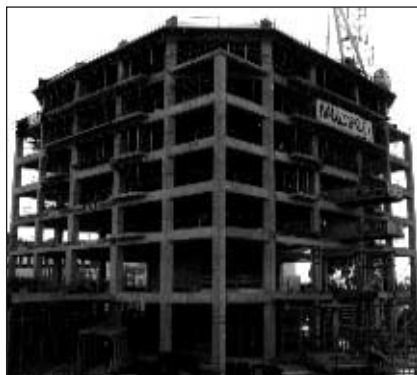
Spencer on Byron building under construction
