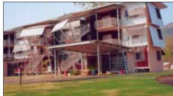
Completed standard 18-unit building with L-shaped floor configuration
