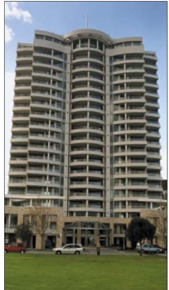
Perth's 18-storey Panorama Apartment complex - the largest totally precast structure in WA
