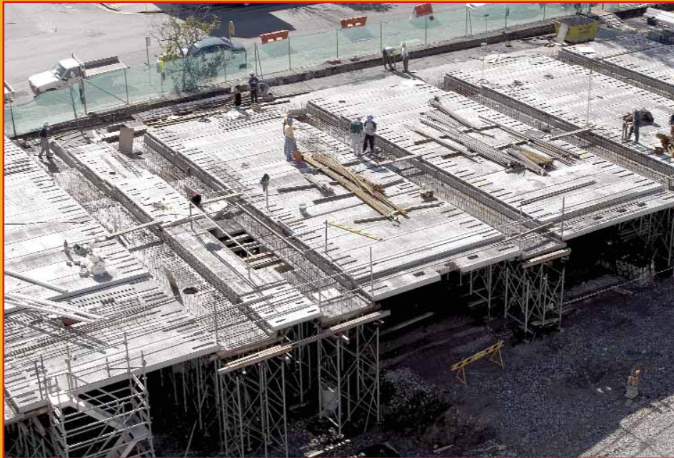
Hollowcore planks span between 2000mm-wide beamshells to form the transfer podium.
