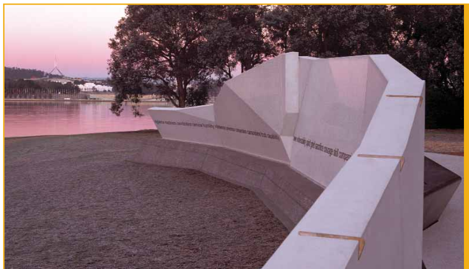
Using precast gave the artist greater scope in designing the six-panel frieze.
