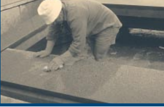
Light acid cleaning of polished panel prior to delivery
