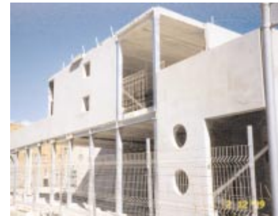
Hollowcore floor planks are installed at the second floor level.
