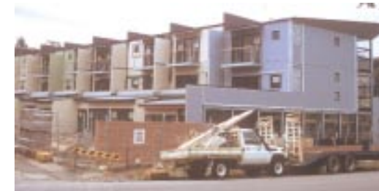
Painting of the panels.
