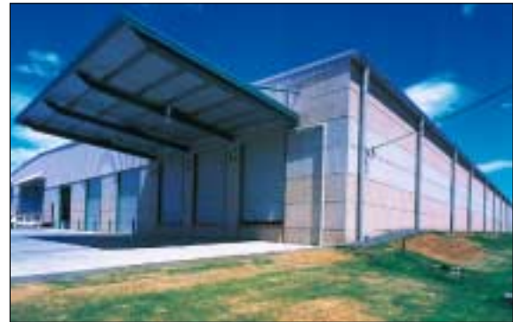
Over 2000 m 2 of fire-rated exposed aggregate hollowcore panels clad this warehouse for Southcorp at Arndell Park, NSW. A banding effect was achieved by using two colours of exposed aggregate.
