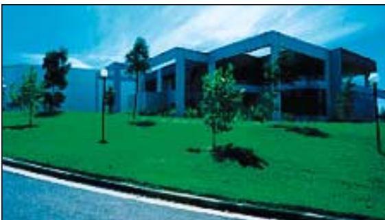
Warehouse in Hallam, Victoria featuring use of precast colonnades, spandrels, and cladding panels coated with a textured paint finish
