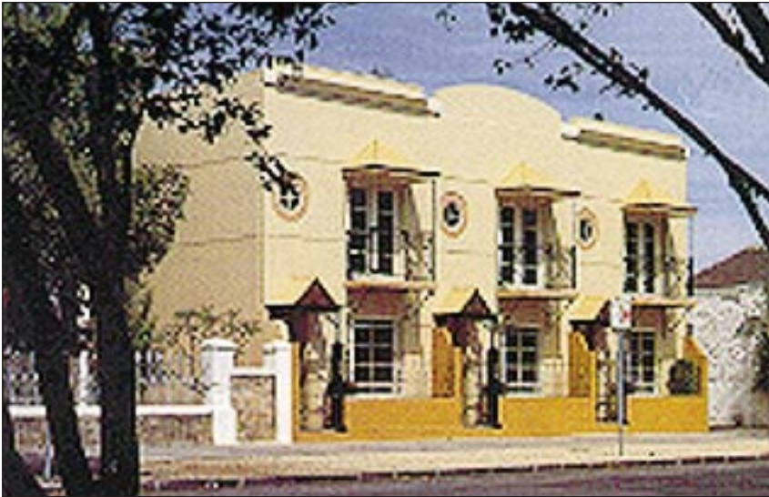
Fully precast, terrace style housing, North Adelaide
