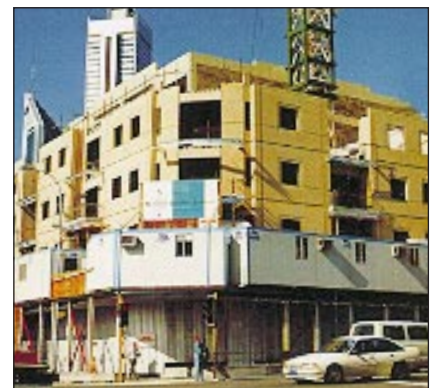
Figure 1 Possible panel configurations. Also 'T', 'L' and 'U'-shaped panels together with spandrel panels alternating with glazing
