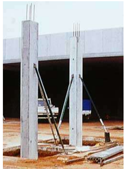
COLUMN POSITIONING AND PROPPING 1
