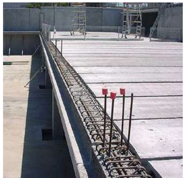
COLUMN TO BEAM CONNECT
