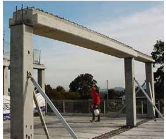
BEAM POSITIONING ON COLUMNS 1
